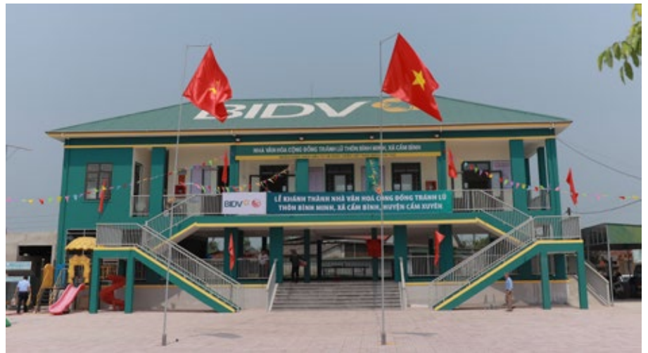
A flood-resilient community house funded by BIDV
