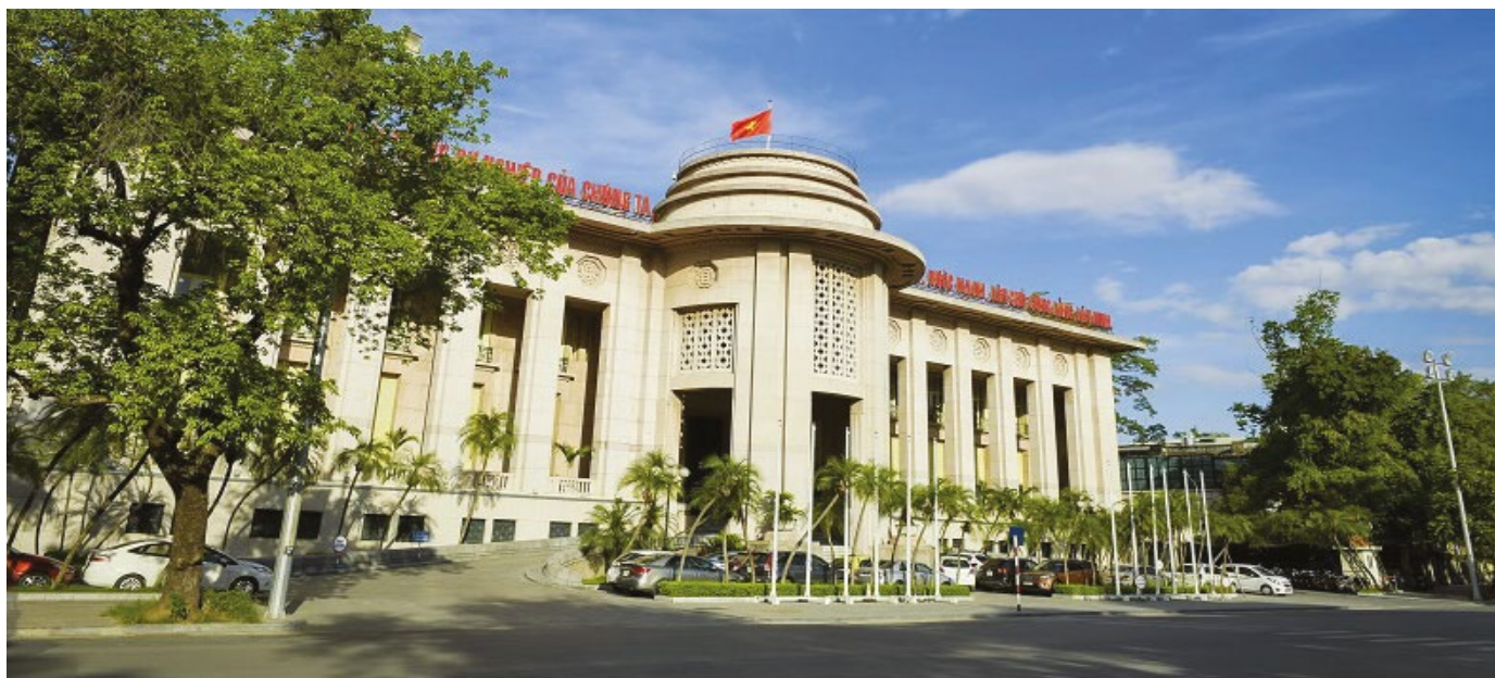
The headquarters of the State Bank of Vietnam
